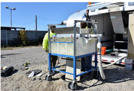
Figure 2. TPU liner threaded through funnel prior to adding grout.
